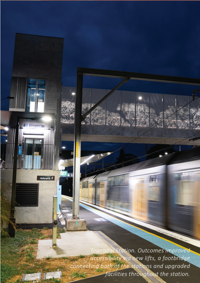
Station entrance at Unanderra incorporating Aboriginal design integration celebrating local Dharawal culture and storytelling.
