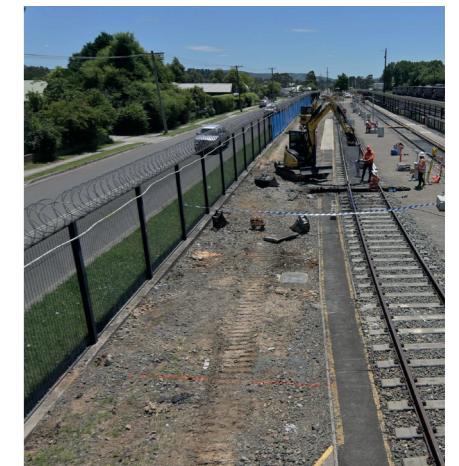
Previous security fencing before being replaced with noise barrier wall.
