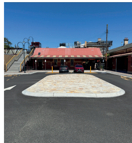
Archaeological sandstone laid by early settlers uncovered during construction was incorporated into the Dalys Way roundabout as a heritage feature.
