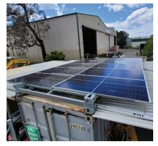
Redeployable Container-Top Solar System at Unanderra Station: In collaboration with Makinex, we developed a solar system mounted on shipping containers to supplement grid energy on construction sites. Paired with battery storage, this innovation has since become a commercially available solution.
